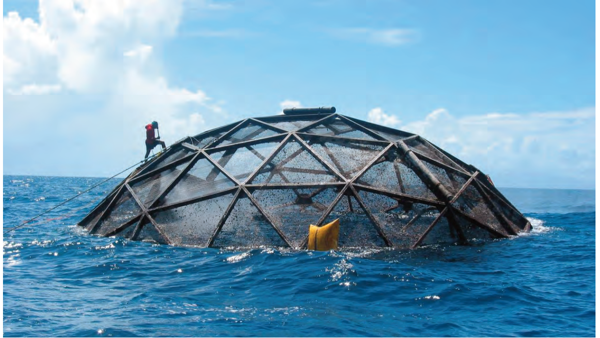
Worker conducting maintenance on a submersible cage
